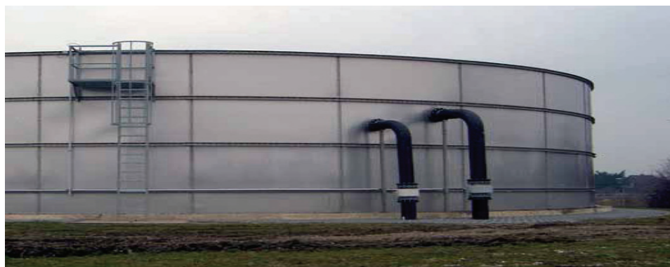
The choice of lean duplex LDX 2404 (R) for a fermentation residue tank in Borken, Germany reduced the weight by 25% in comparison to a 316 type stainless steel tank. Photo: by courtesy of Börger GmbH, Borken-Weseke, Germany.
