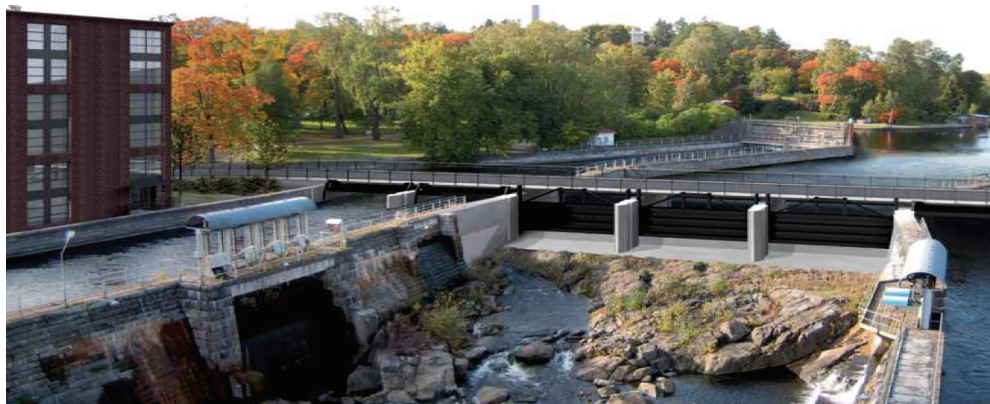
The use of light yet high strength duplex for sluice and flood gates in a Finnish hydropower project enabled material savings and meant less hydraulic force was needed to operate the gates.
